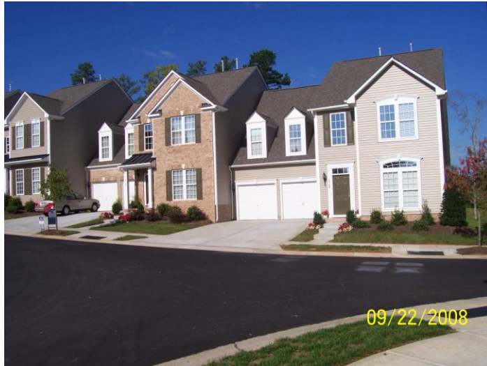
Acceptable two single bay front loading garages
