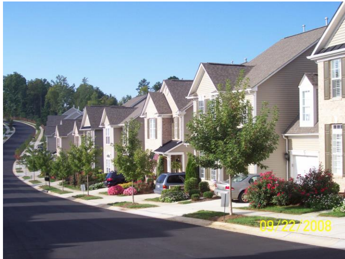
Acceptable recessed double bay front loading garages
