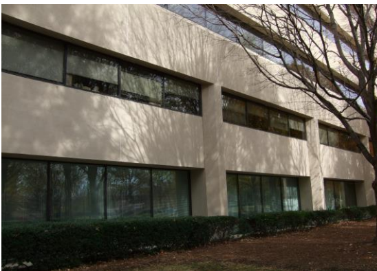
Figure 3 – Continuous ribbon windows
